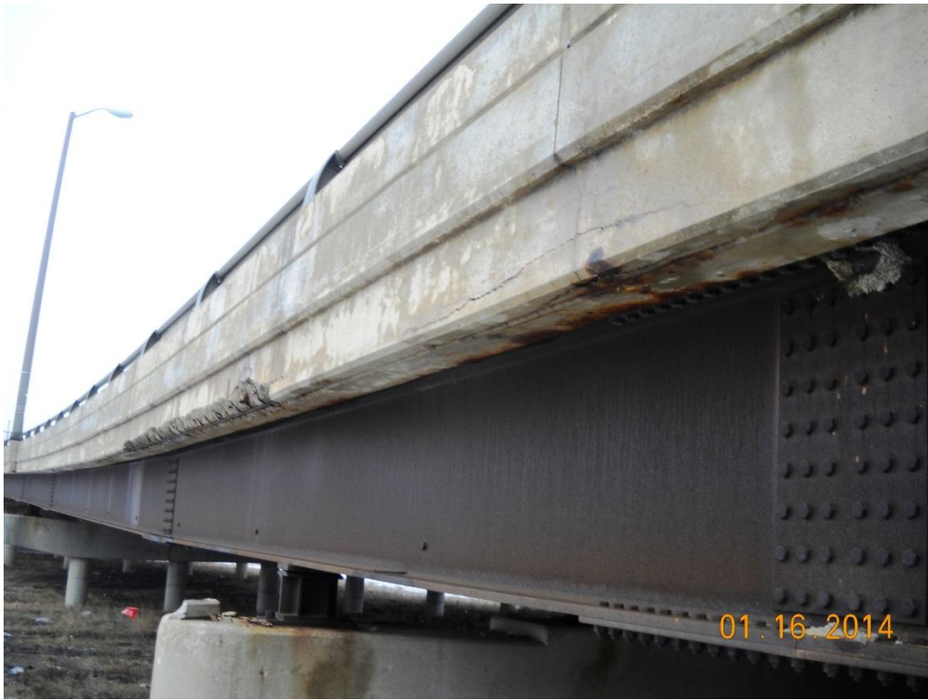
Photo No. 28 West deck fascia – typical condition, looking SW
