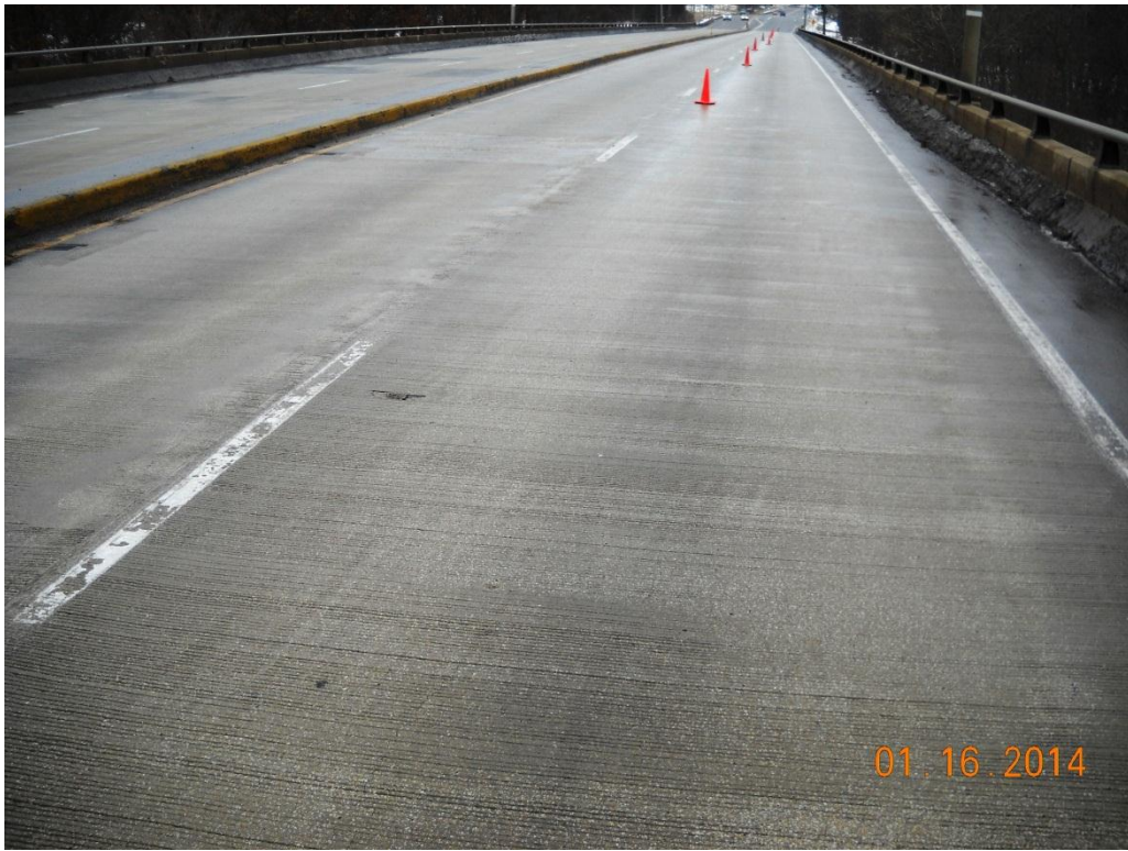
Photo No. 20 Top of deck, span 9 SB, looking south
