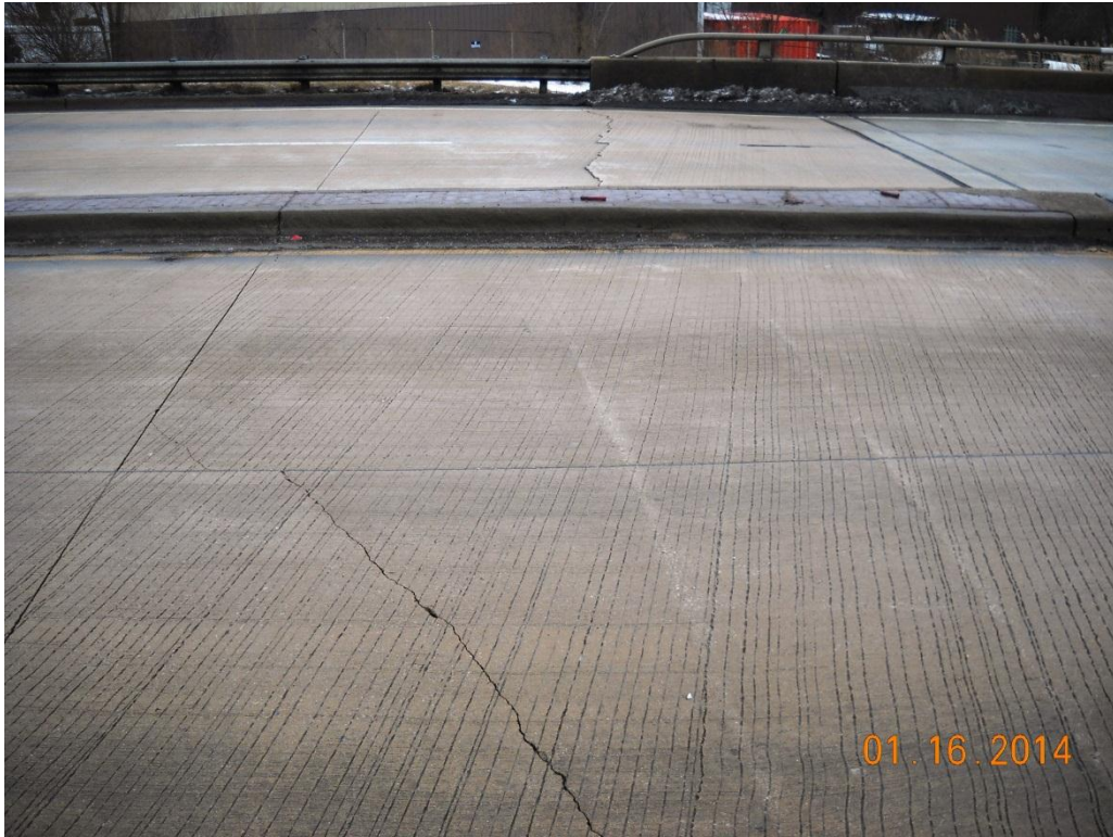
Photo No. 7 North approach pavement looking east
