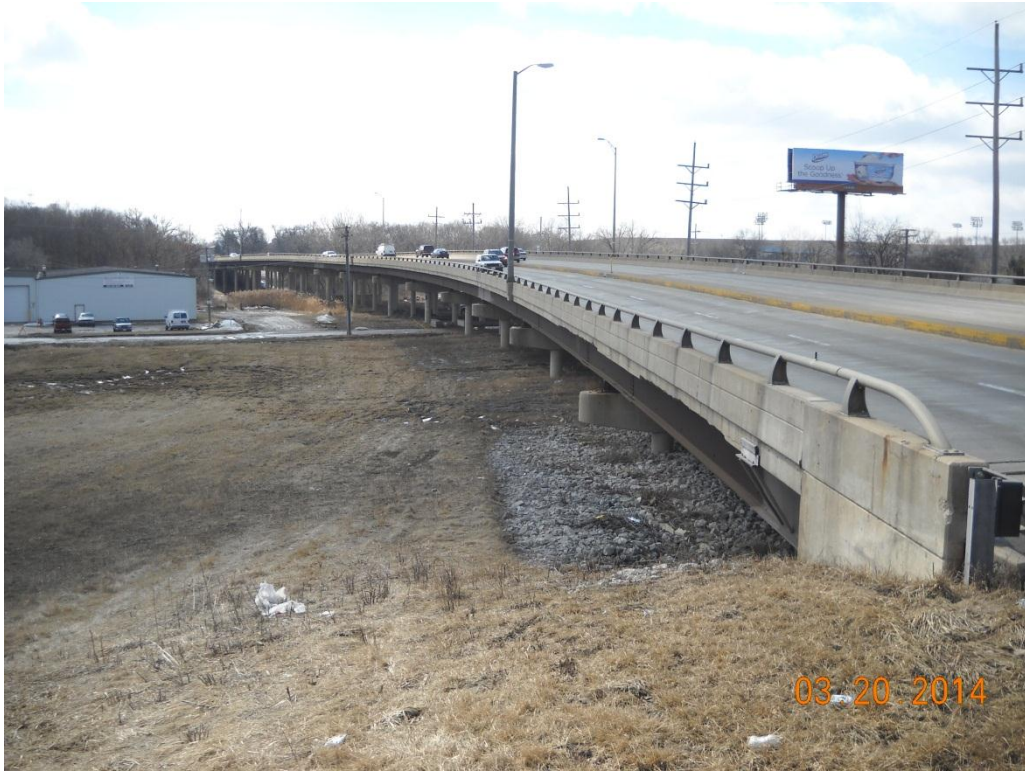
Photo No. 5 East elevation of bridge
