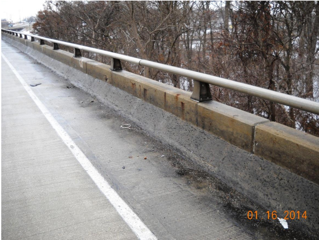
Photo No. 15 East parapet looking northeast
