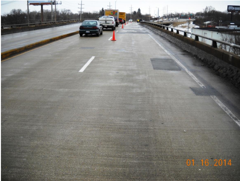
Photo No. 23 Top of deck, span-8 NB, looking north
