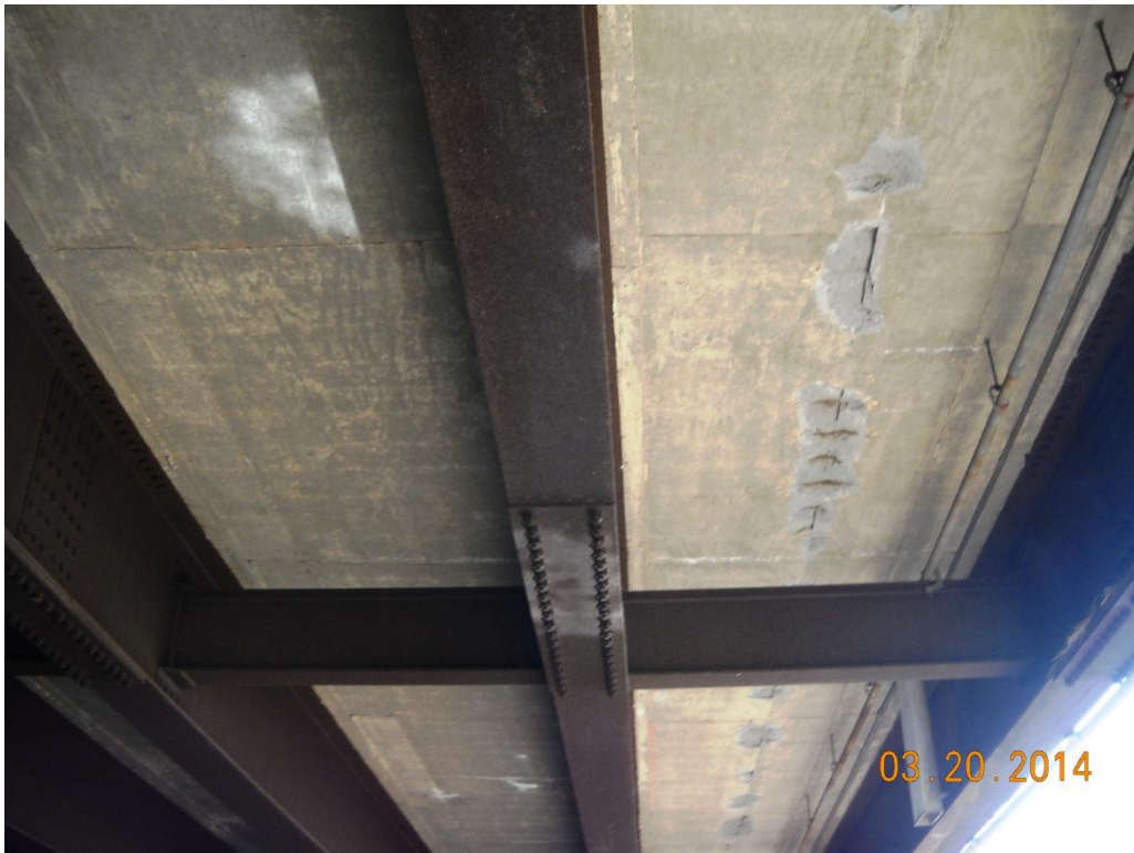
Photo No. 33 Fascia bay - typical
