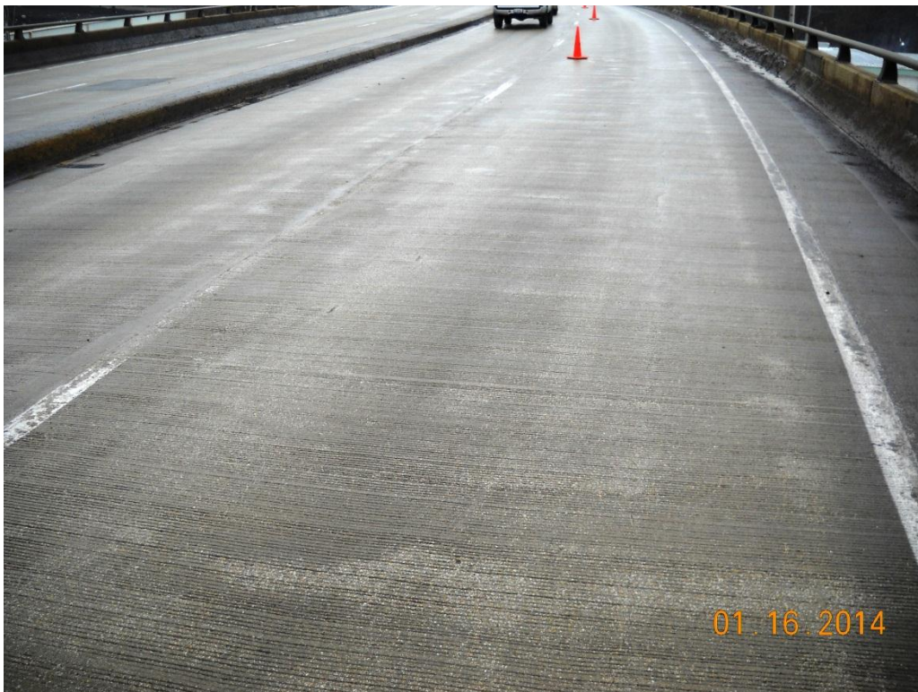
Photo No. 18 Top of deck, span 5 SB, looking south
