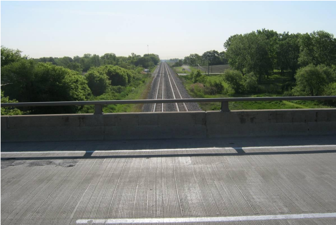
Photo No. 3 Looking east from bridge (2012 photo)
