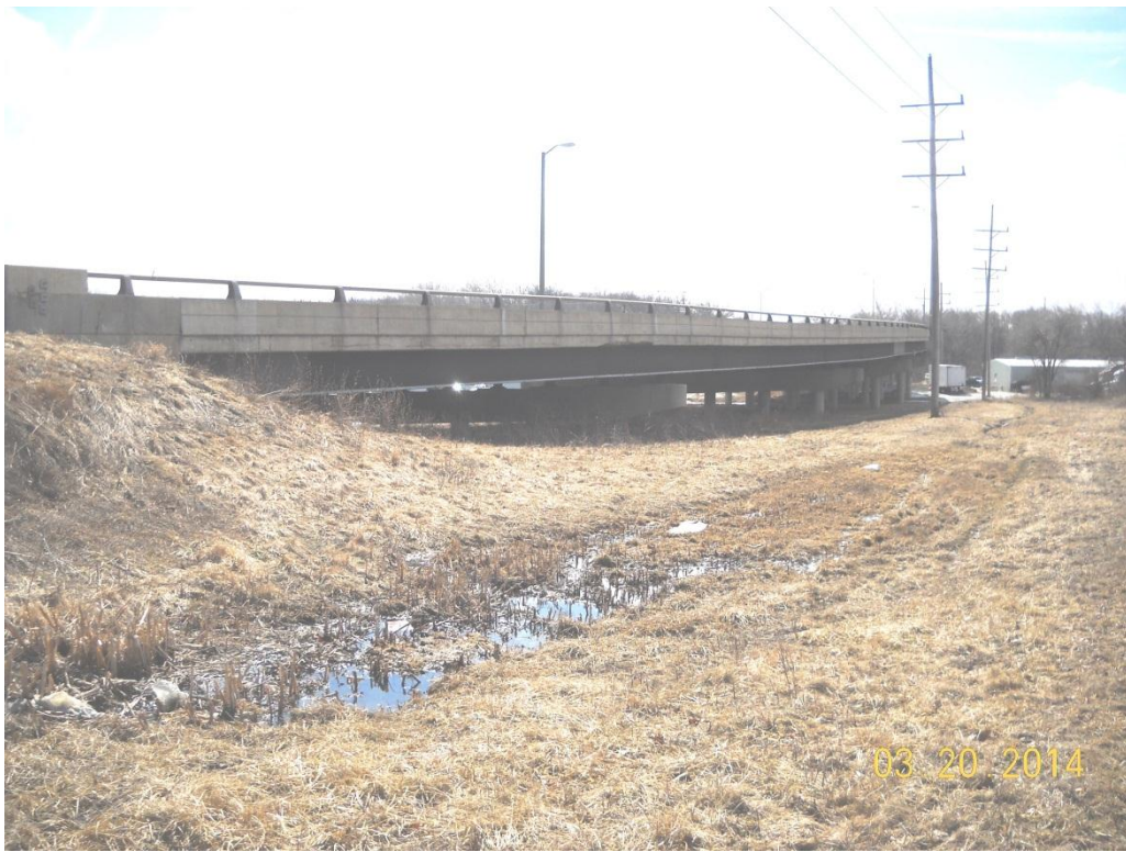
Photo No. 6 West elevation of bridge
