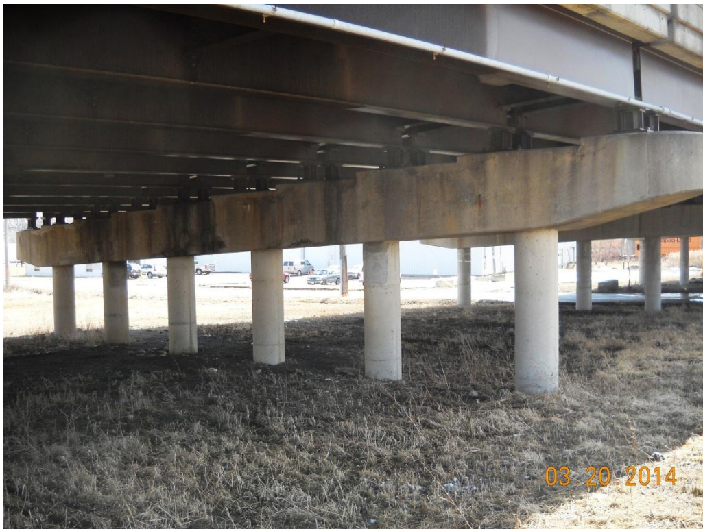
Photo No. 44 Pier 3, looking SE
