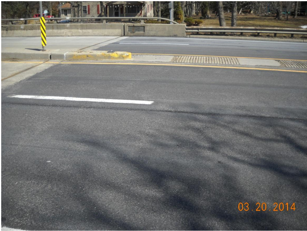
Photo No. 8 South approach pavement looking east
