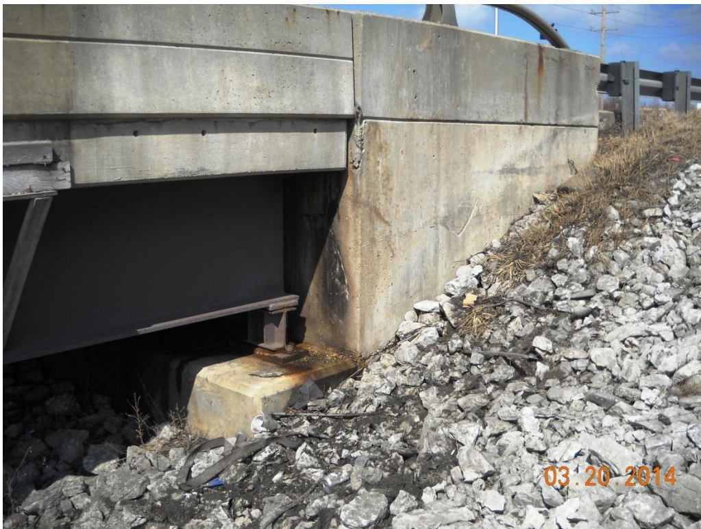
Photo No. 42 NE abutment wingwall
