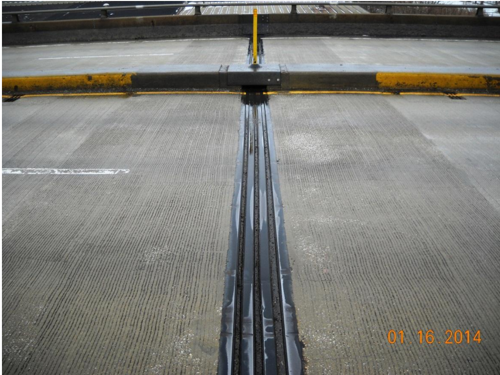
Photo No. 11 Pier 8 transverse joint
