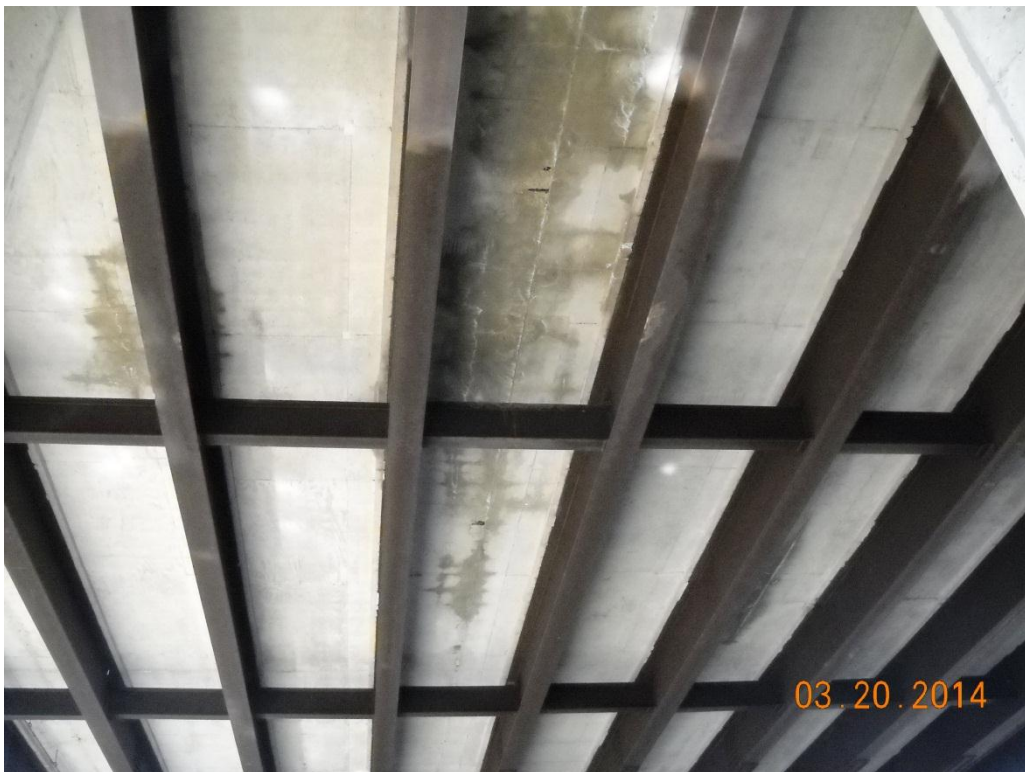
Photo No. 34 Bottom of deck and beams, span-13, looking north
