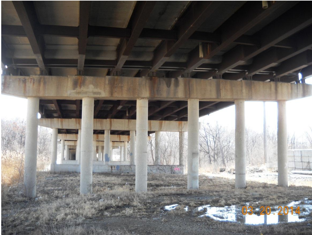
Photo No. 47 Pier 8, looking south
