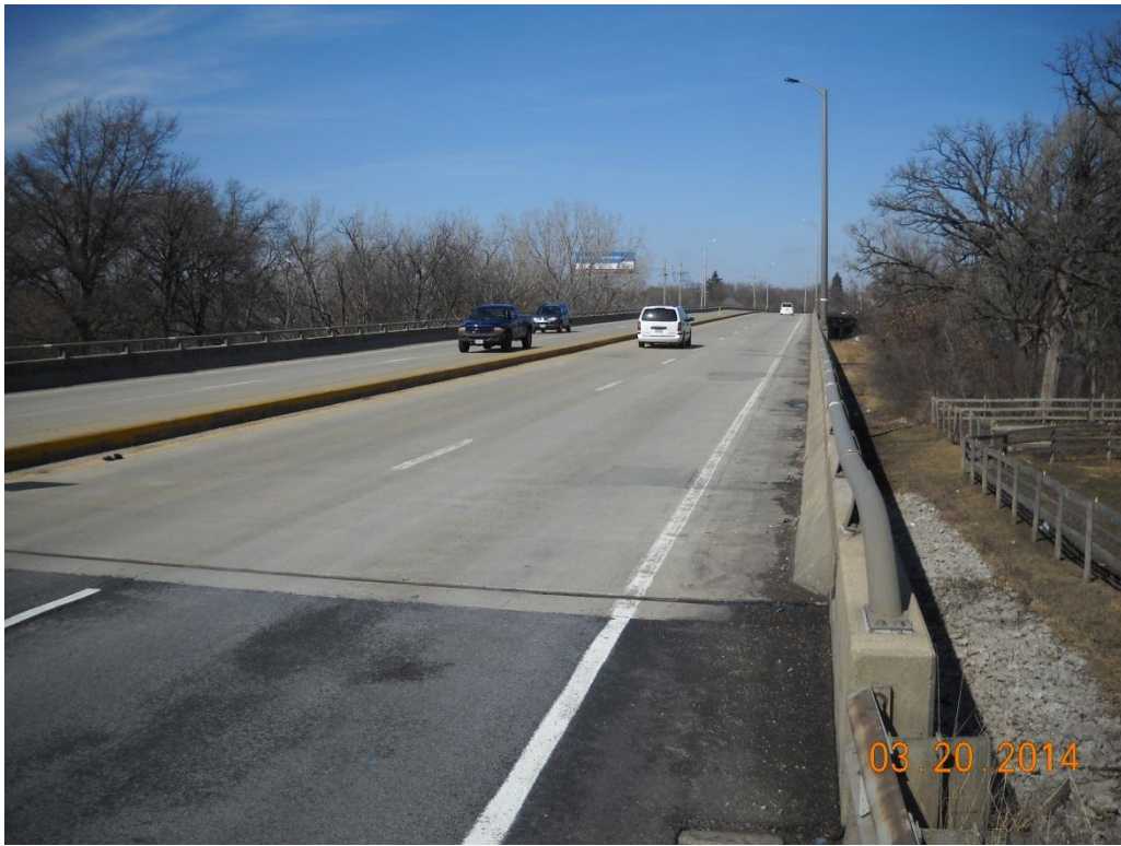
Photo No. 2 Looking north through bridge
