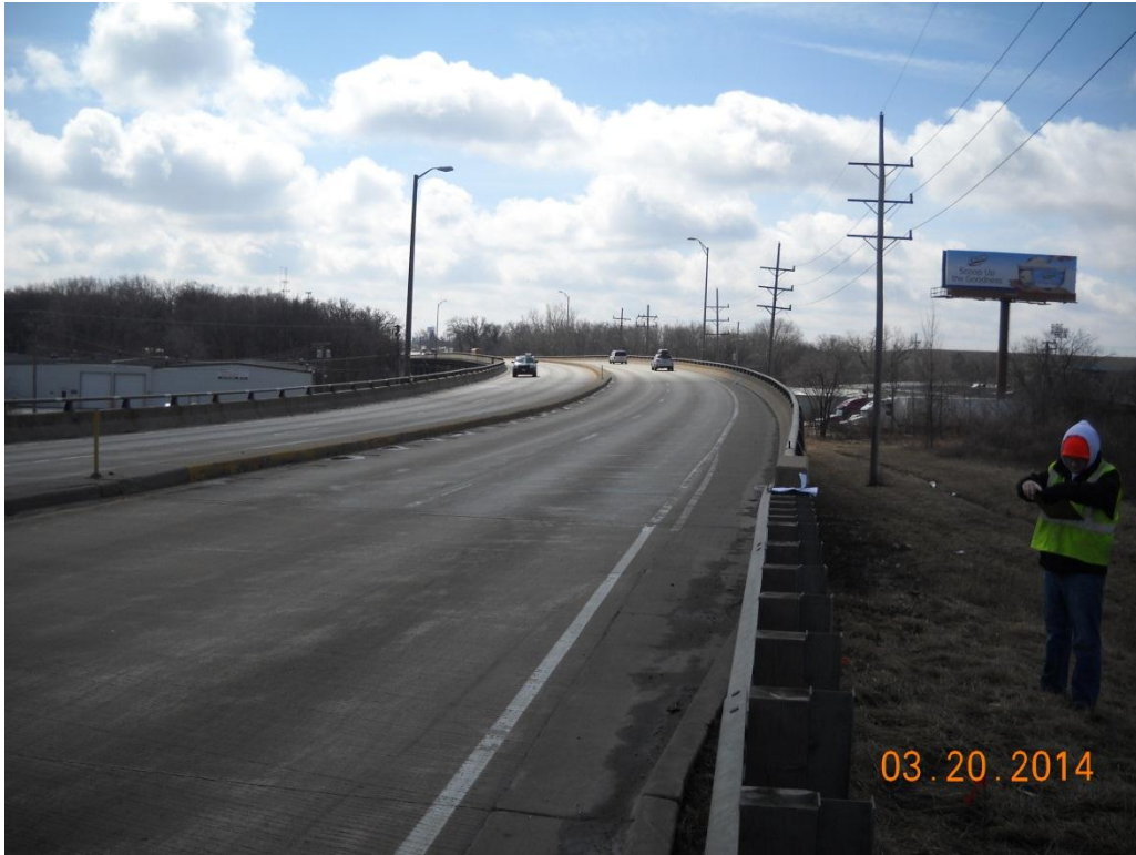
Photo No. 1 Looking south through bridge
